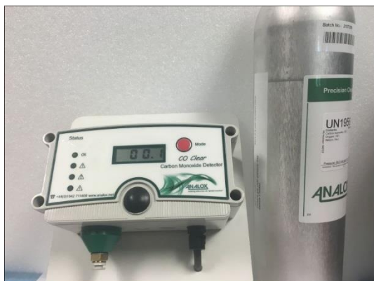
Connecting of the gas cylinder
